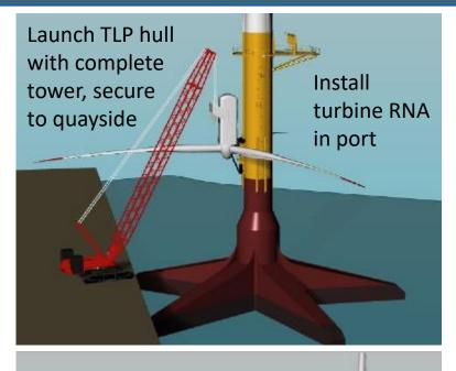
Float out with one tug, stabilized by RNA at bottom position
