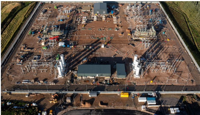
Moray West onshore substation during construction near Keith, Moray
