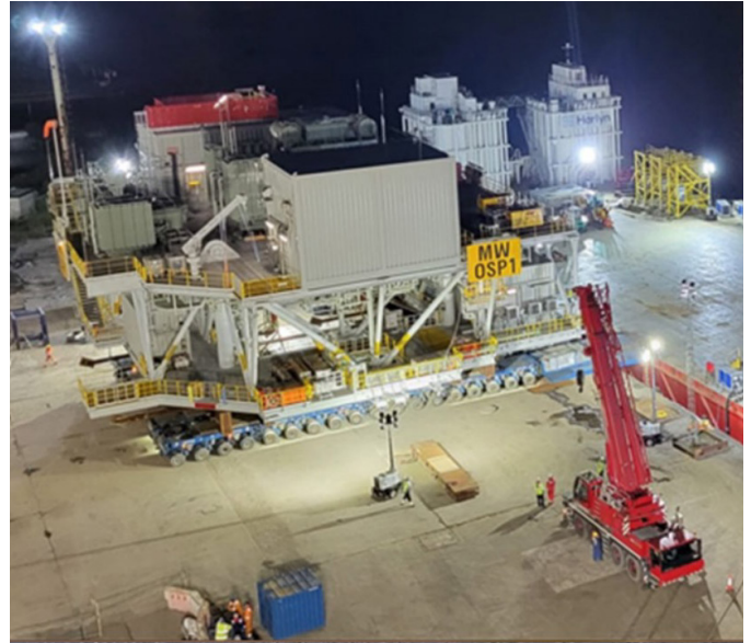
Load-out of completed offshore substation, destined for Moray West
