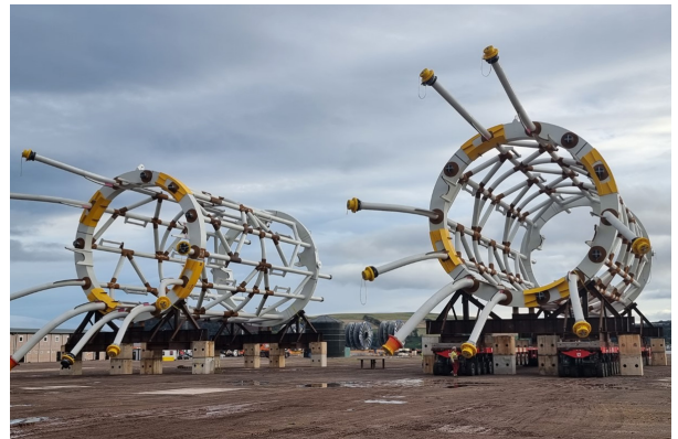
J-tube cages in GEG's fabrication shop at Port of Nigg
