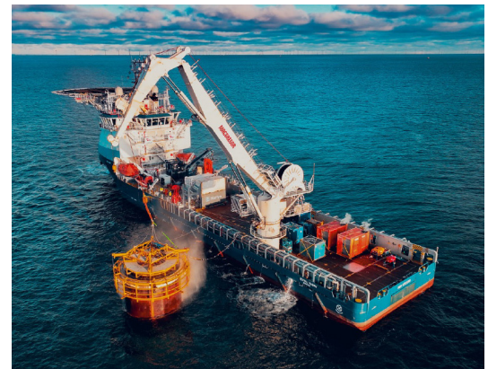
Harlyn were contracted for the monopile cleaning using the Claxton tool
