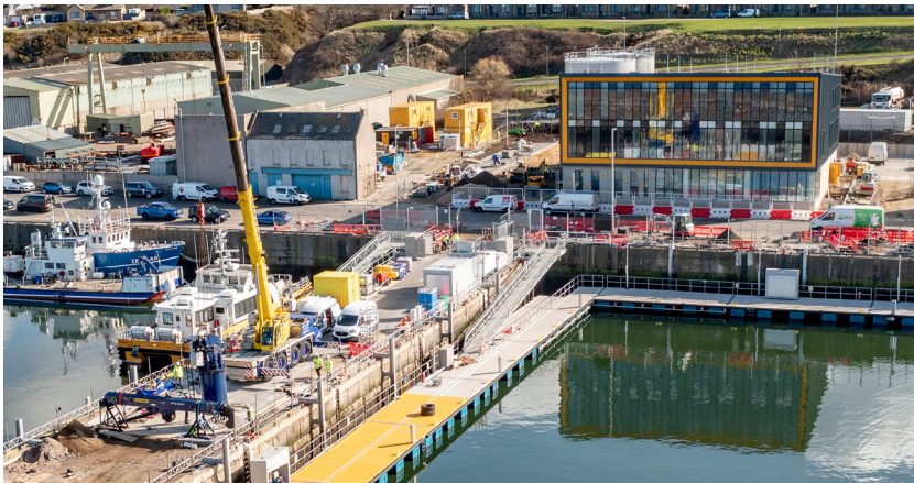
Operations base in Buckie during construction
