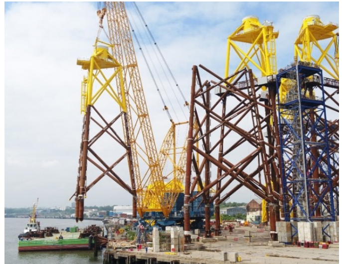
Jacket foundations for Moray East being loaded out of Smulders UK
