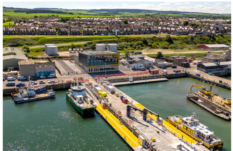
Buckie O&M Base and harbour upgrades, June 2024
