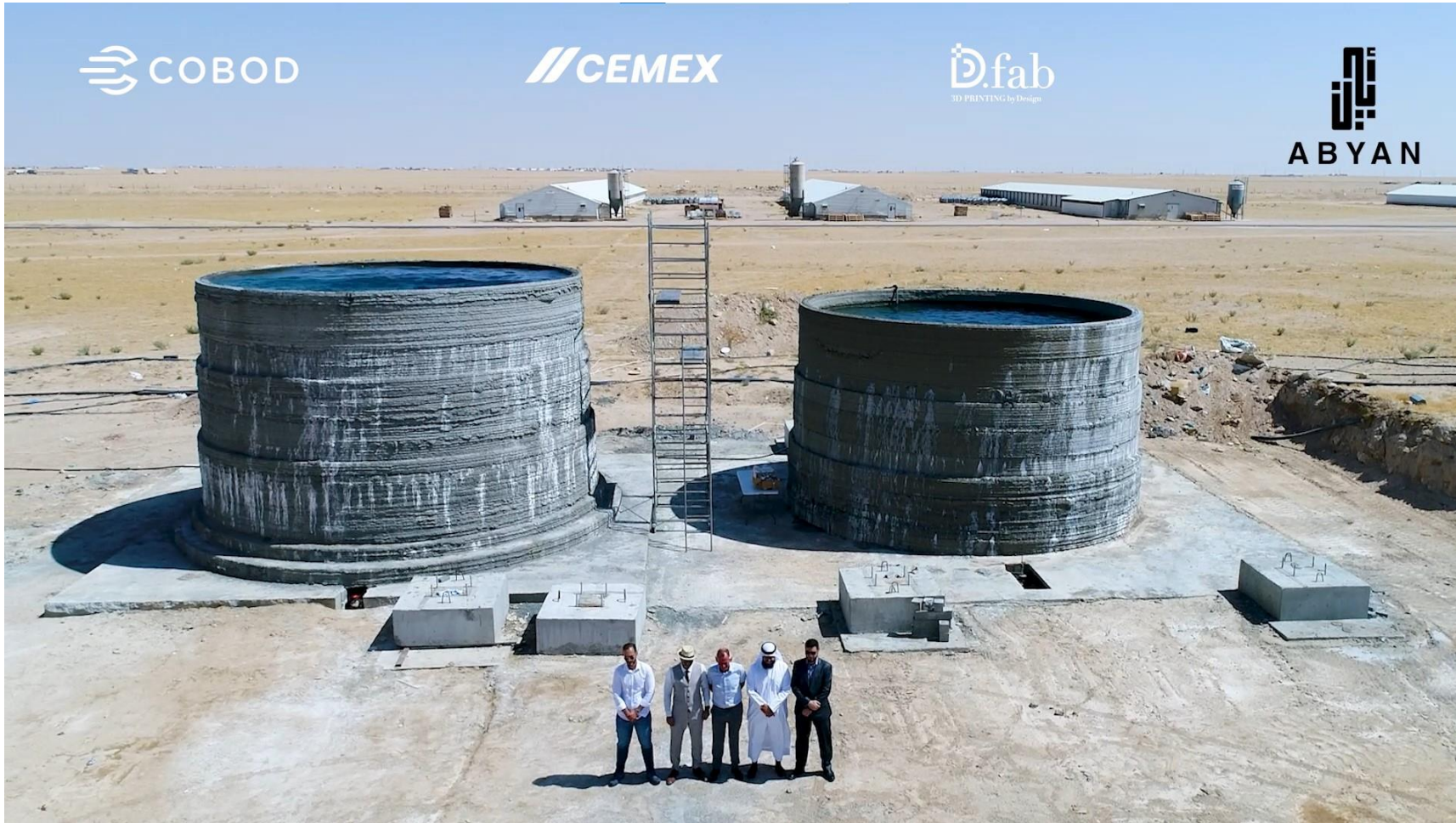
2 chicken drinking water tanks, 4,5m tall and 7m diameter. Kuwait.
