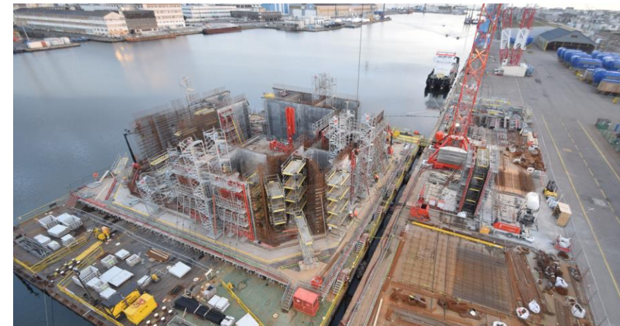
Floatgen floating foundation construction (2016)
