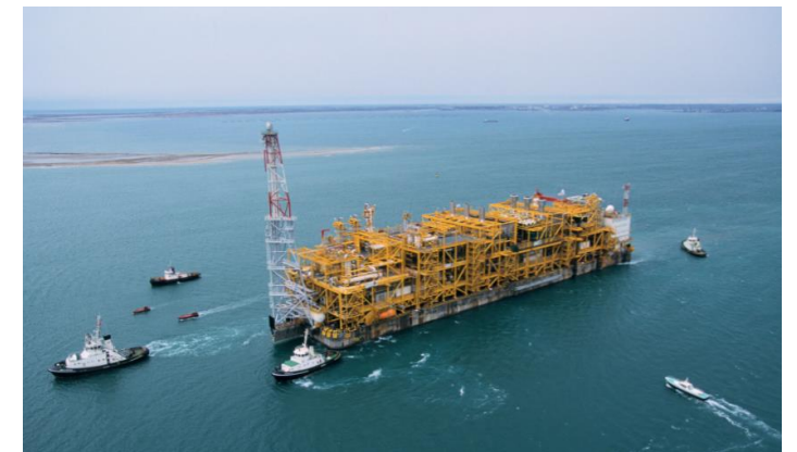
N'kossa concrete floating barge (1994)
