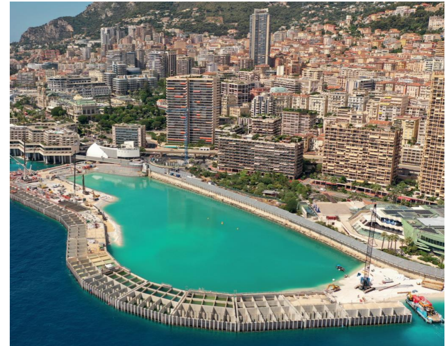
Monaco port extension – Concrete caissons (2020)
