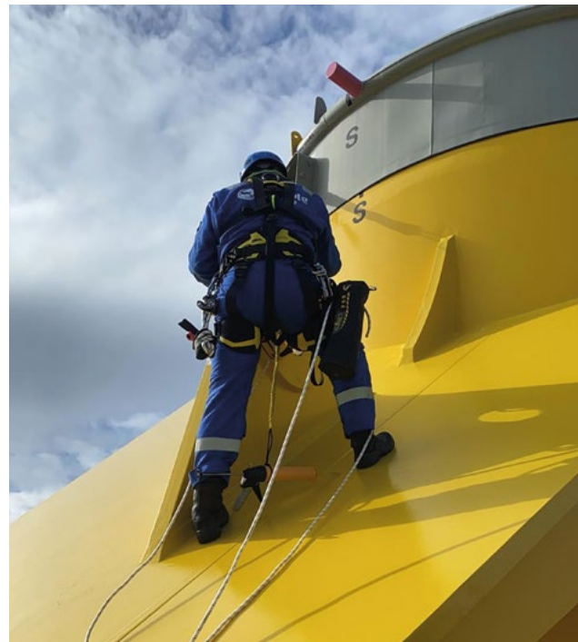
Rope Access Painting in Moray East Offshore Wind Farm
