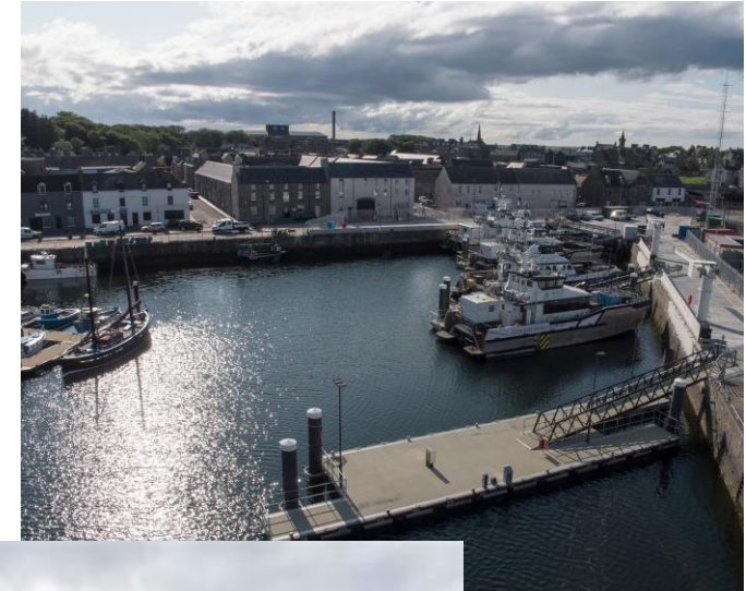
Beatrice (Wick) – renovation of existing historic buildings
